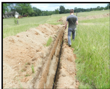
Water pipeline installation for livestock
