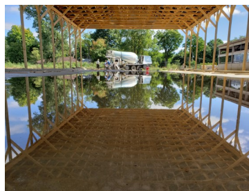
Manure Dry Stacking Storage Facility (during final concrete pour, and after wall installation) - allows storage of animal waste during winter months, eliminating need for winter spreading thus reducing runoff contamination
