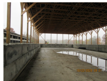
Manure Dry Stacking Storage Facility (during final concrete pour, and after wall installation) - allows storage of animal waste during winter months, eliminating need for winter spreading thus reducing runoff contamination
