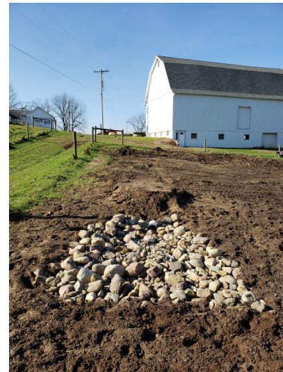
Underground outlet from new gutters diverts runoff away from feeding areas
